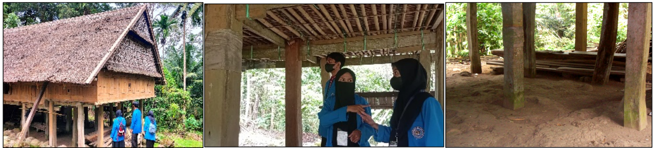
Figure 3. Components of the Karampuang Traditional House
